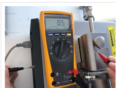
Checking the resistance between the reactor chamber and the ground point.
